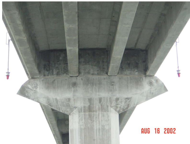
Figure 2. Superstructure of Humboldt Bay Middle Channel Bridge.
